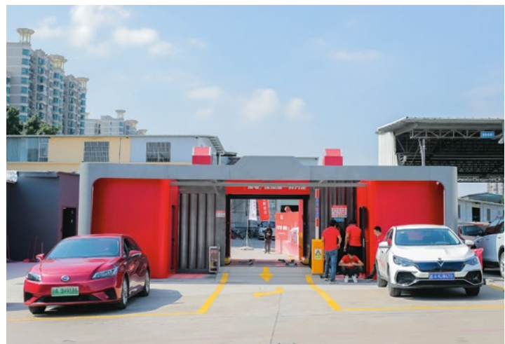
Aulton Dianba Batteriewechselstation 4.0
